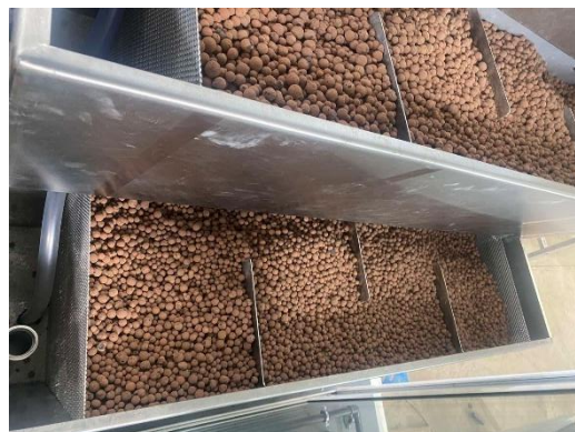
Figure 65 vertECO® modules filled with substrate to begin plantation
