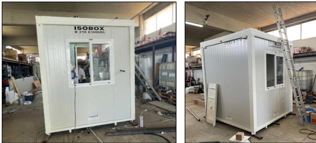
Figure 75 Side Views of the Isobox Frame during Construction
