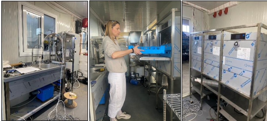
Figure 61 The basin (left), staff position (middle) and dishwashing units (right) inside the large-scale unit. Given the substantial quantity of items requiring washing, it is apparent that the container lacks adequate drying space. Furthermore, for reasons of hygiene and operational efficiency, it is crucial to distinctly separate soiled and cleaned items. Consequently, the incorporation of external areas or on-site tents is being considered from the outset.
